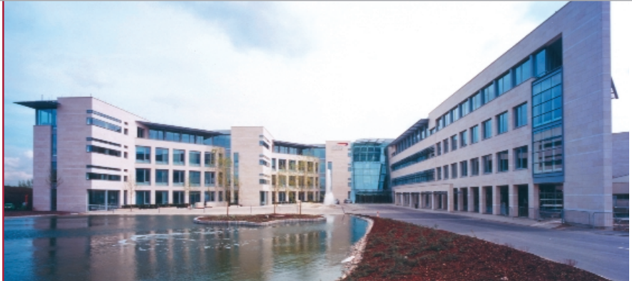
The British Airways Headquarters near London, England, offers occupants the convenience of working, shopping and dining under a common roof.
